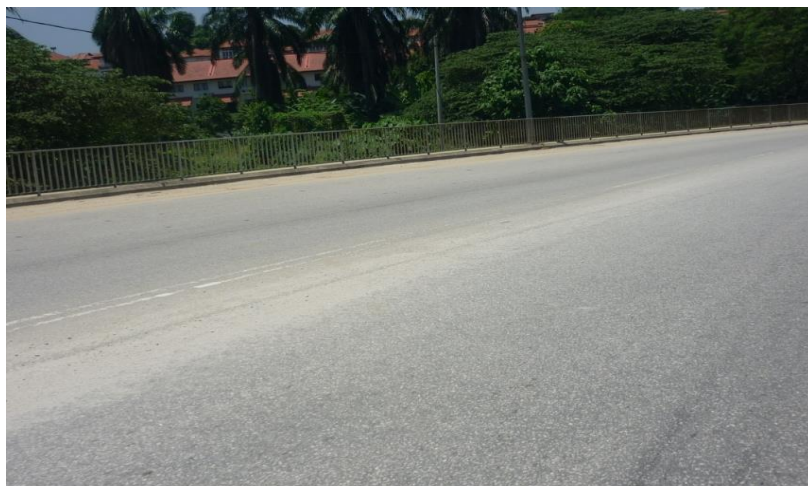
Rajah 18 : Faded Road Marking
