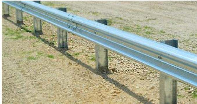
Rajah 35 : Double Rail Guardrail
