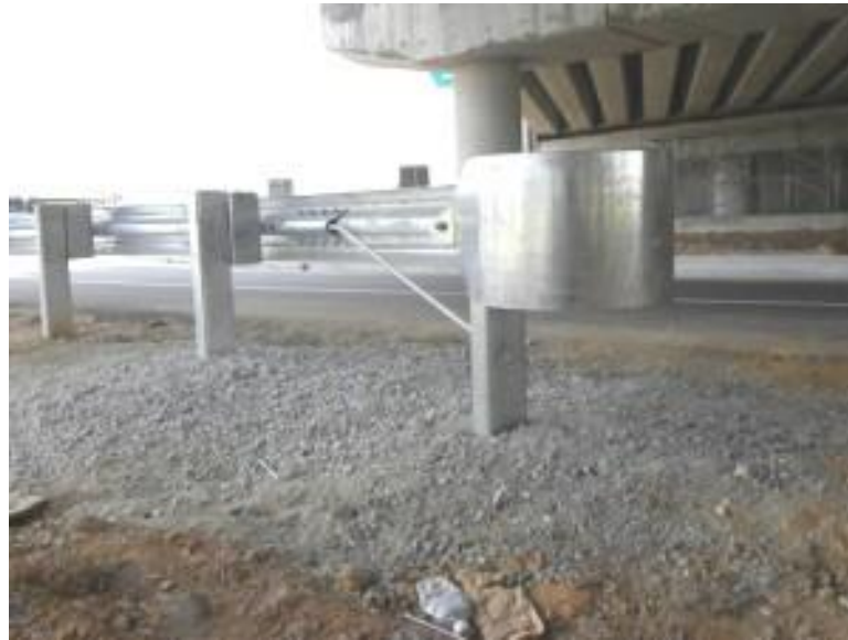
Rajah 39 : Terminal Anchorage Unit
