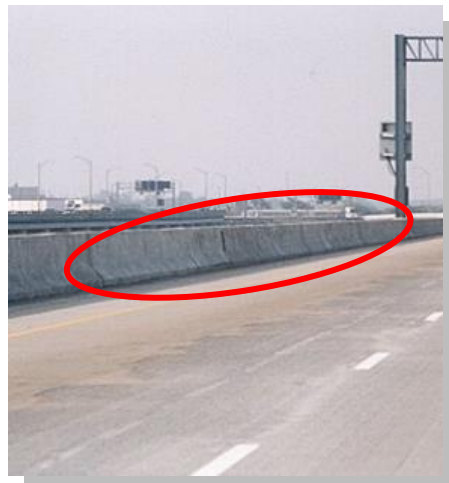
Rajah 32 : New Jersey Barrier
