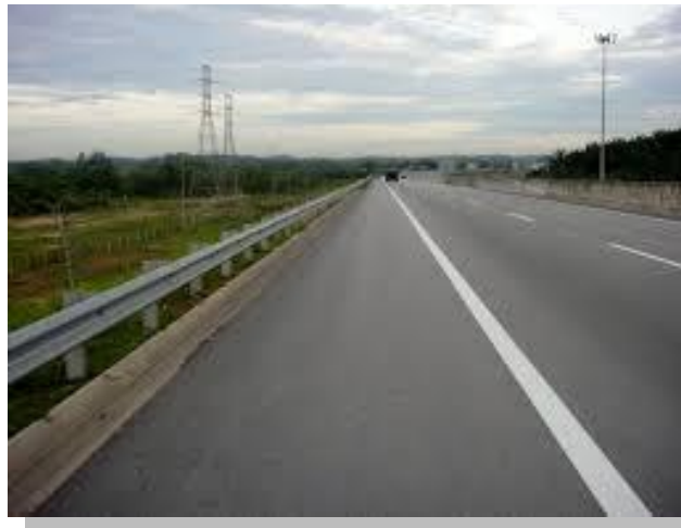
Rajah 6 : Shoulder paved / berturap
